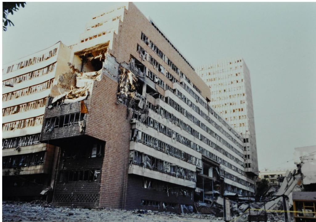
**Figure 9.** Building B after the first bombing, visible damage to the cascading part of the building towards Nemanjina Street, as well as the destroyed entrance pavilion. May 1999. Author: Dragiša Poznanović
