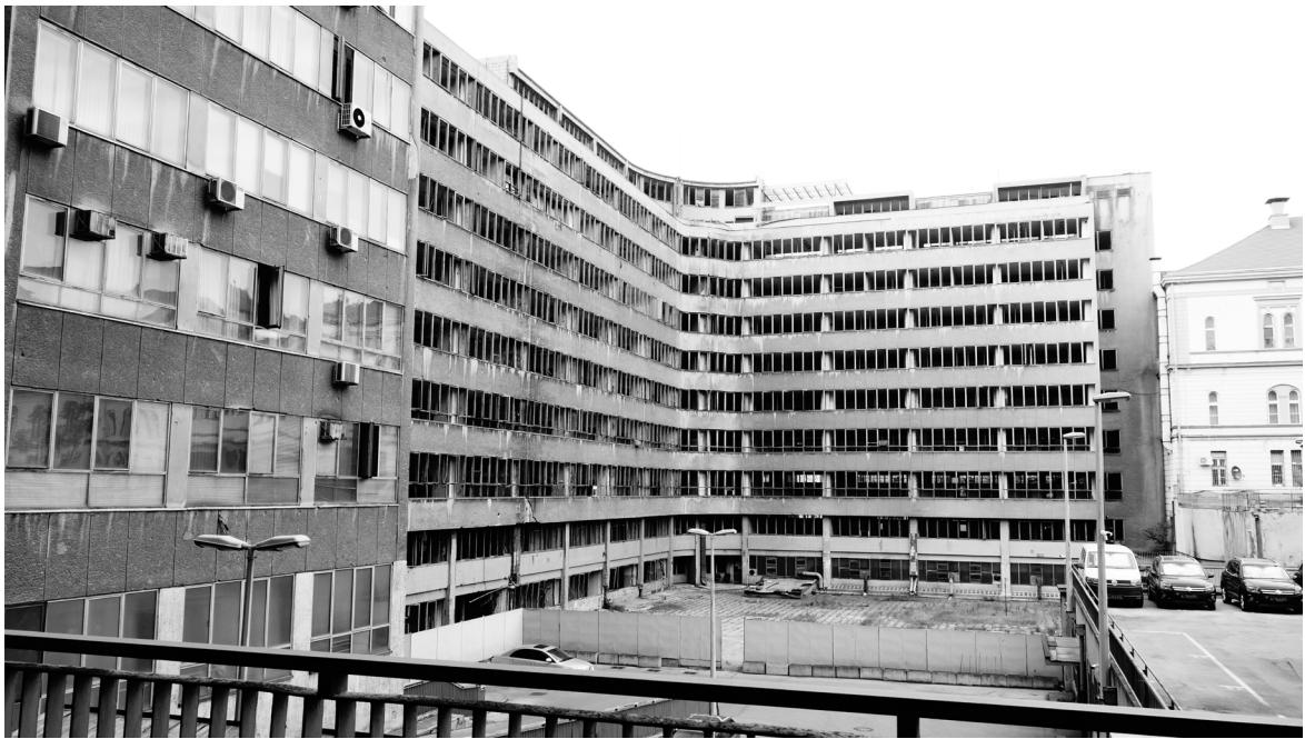
**Figure 10.** Building B, facade of the building from the inner courtyard, windows shattered from the detonation during the second attack. Photo taken in November 2020. Author: Vladana Putnik Prica
